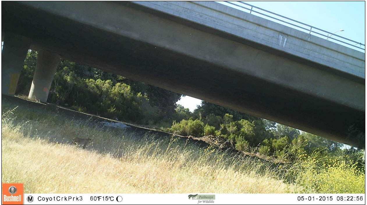
Figure 4. Bobcat traveling under the Bailey Overpass 5-1-2015.
